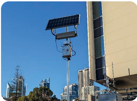
Black Carbon Module at RAC West Perth Head Office
